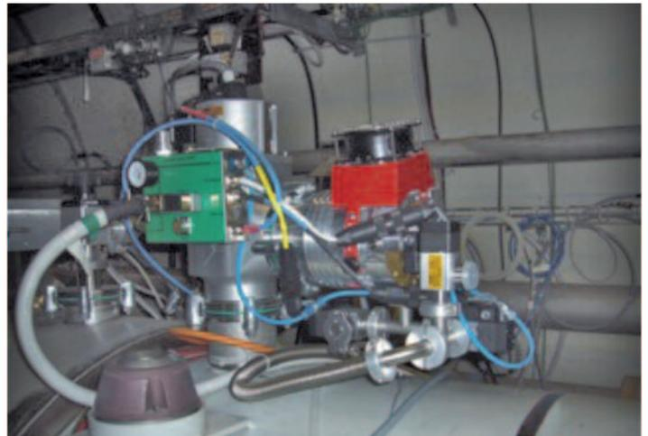
Insulation vacuum generation with HiPace 300 turbopump
