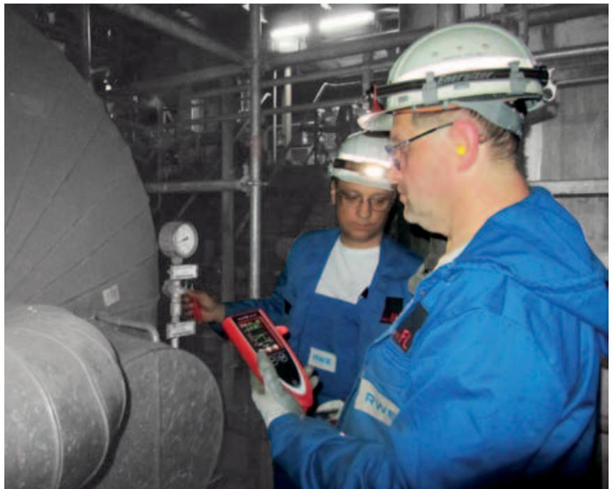
Checking the leak rate on a low-pressure pre-heater with the MiniTest 300. Measured values are indicated on the wireless remote control.
